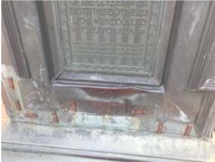
Detail of damage to copper trim
